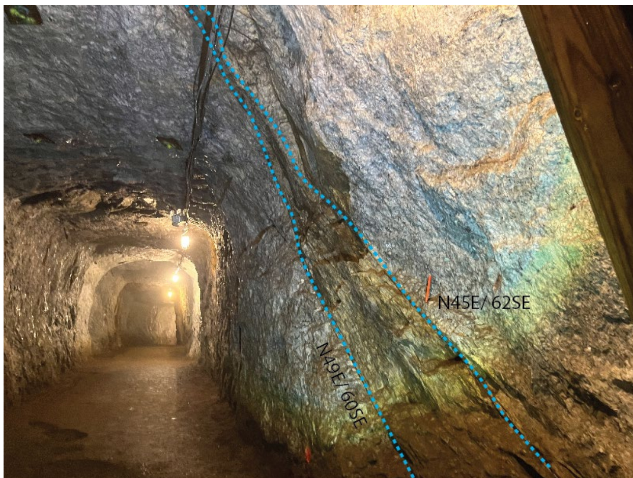
Figure 10. Mylonitized marble in front of the timber sets, which belongs to the set 1 group of faults described in chapter 3 of this volume.
