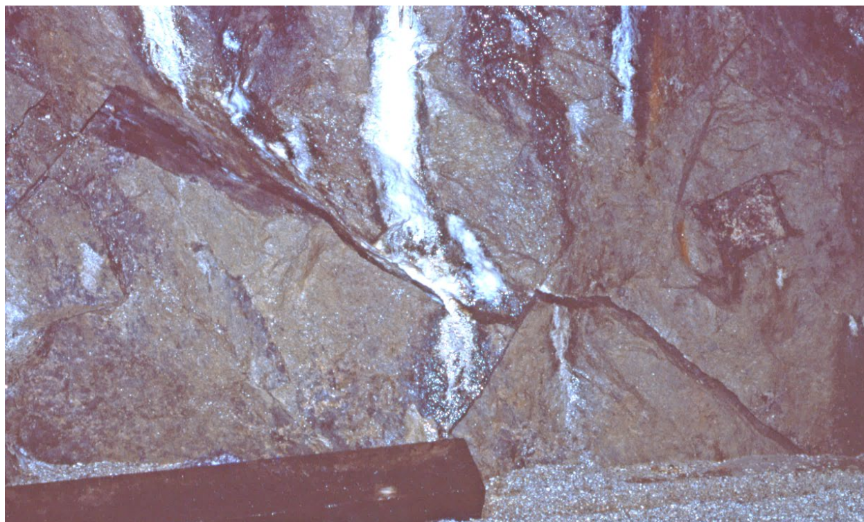
Figure 5. Crosscutting faults (to right of center) in the Sterling mine. The white deposits are calcite flowstone deposited by infiltrating water. For scale, the square plate of the rock bolt at right is about 5 inches on edge.
