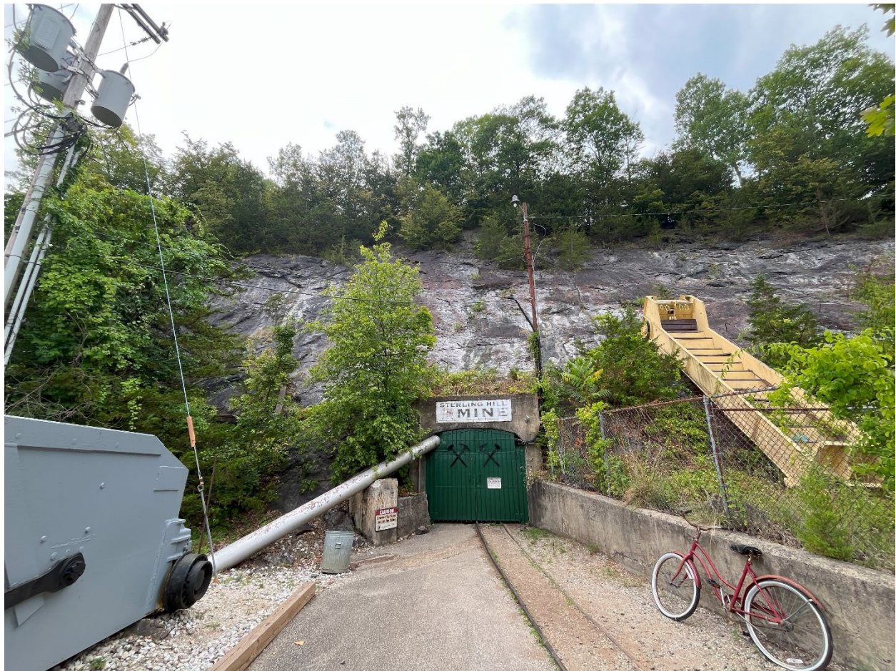
Figure 3. The green doors cover the mine portal. Water and compressed air pipes can be seen on the left. A yellow man car that used to shuttle miners to their workstation sits at right
