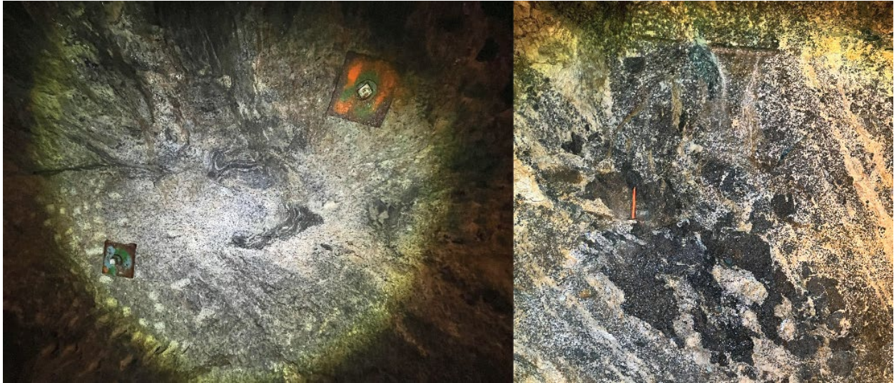
Figure 18. Marble exhibiting fluidized flow patterns hosting blocks of gneiss are visible in certain sections of the Landmesser tunnel.
