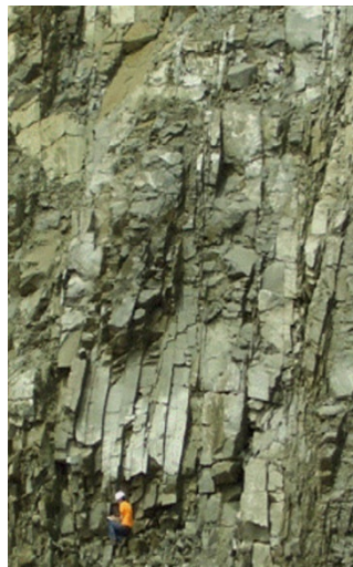
Figure 1a. Photograph of the Stockton Formation depicting bedding plane partings and two sub-orthogonal joint sets (photo from NJDEP)
