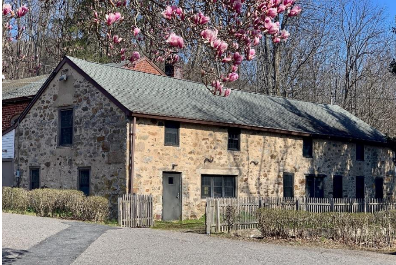
Figure 1. Former Bowers Iron Foundry Building made of Hardystone quartzite locally quarried and from field stones.
