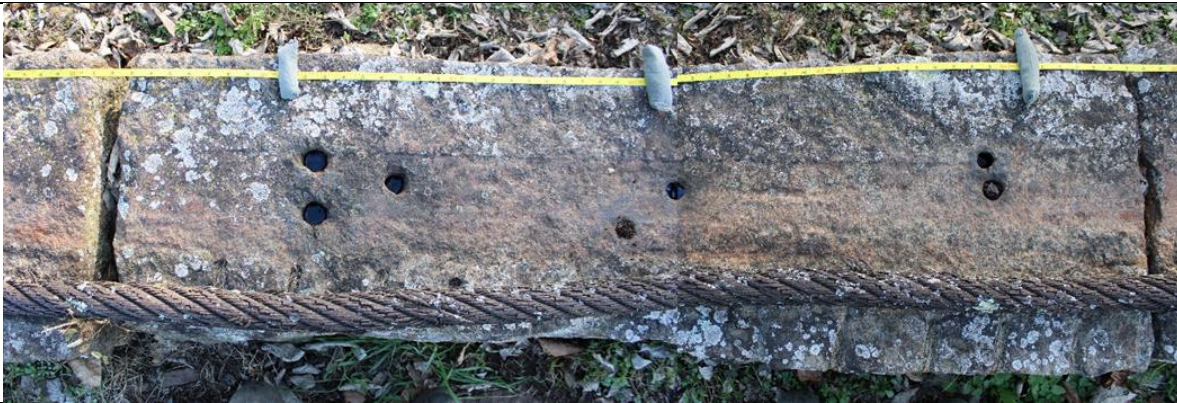
Figure 8. Single stone sleeper that is more than 5 ft. long.
