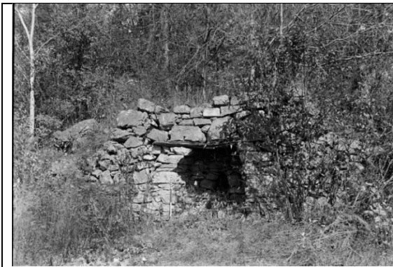
Figure 1A. Small limestone kiln to convert limestone to cement and lime.
