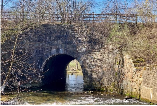
Figure 4. Aqueduct to permit Pequest stream to flow under Morris Canal.
