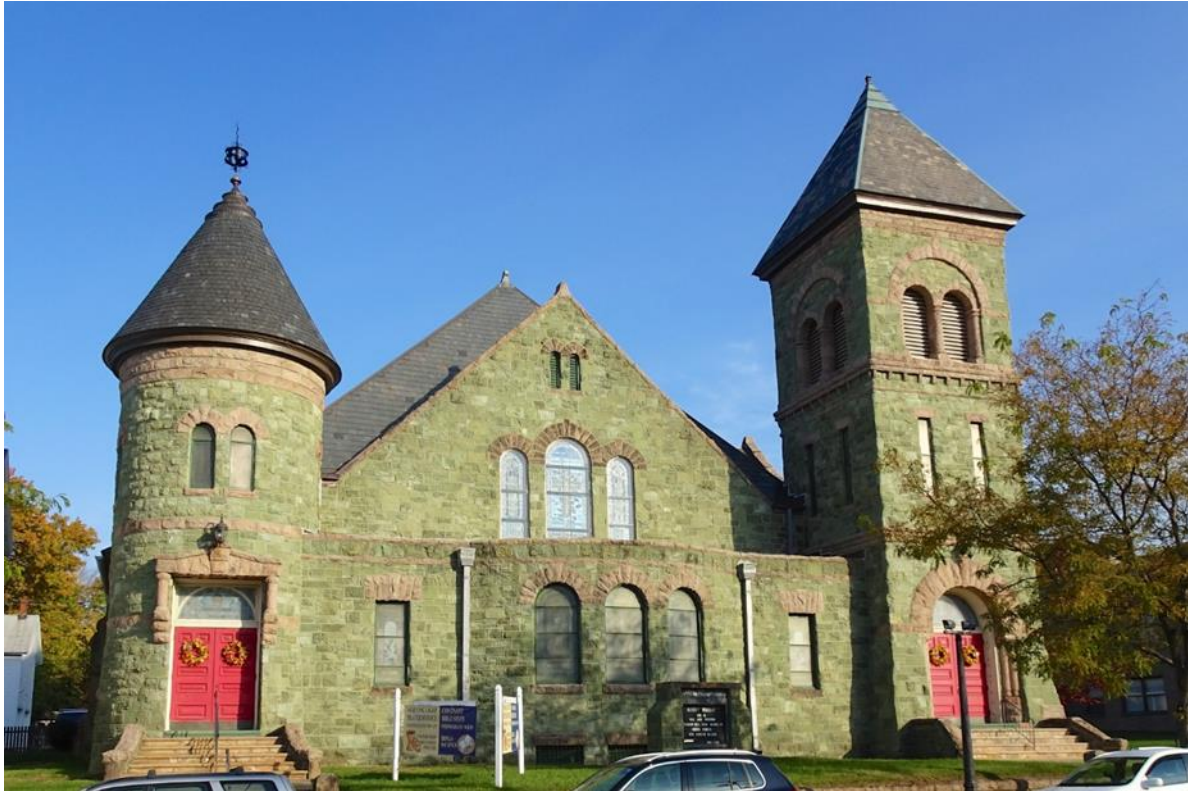
Figure 1. First Methodist Episcopal Church, Washington, NJ. built 1895-98. Stone used includes serpentine (green), sandstone (pink), and slate (roof).
