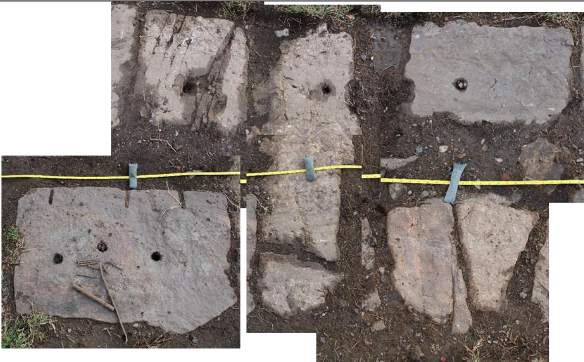
Figure 9. A series of stone sleepers with one sleeper that supported rails for both Rows B and C.
