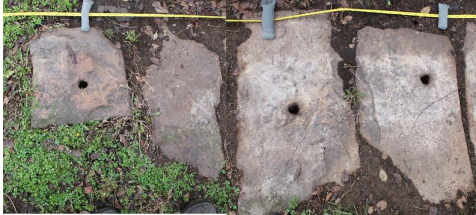
Figure 7. Four stone sleepers with one that is less than 1 ft. long.
