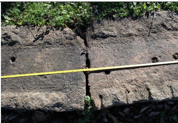
Figure 10. Wide Chiseled Groove on top surface of stone sleepers.
