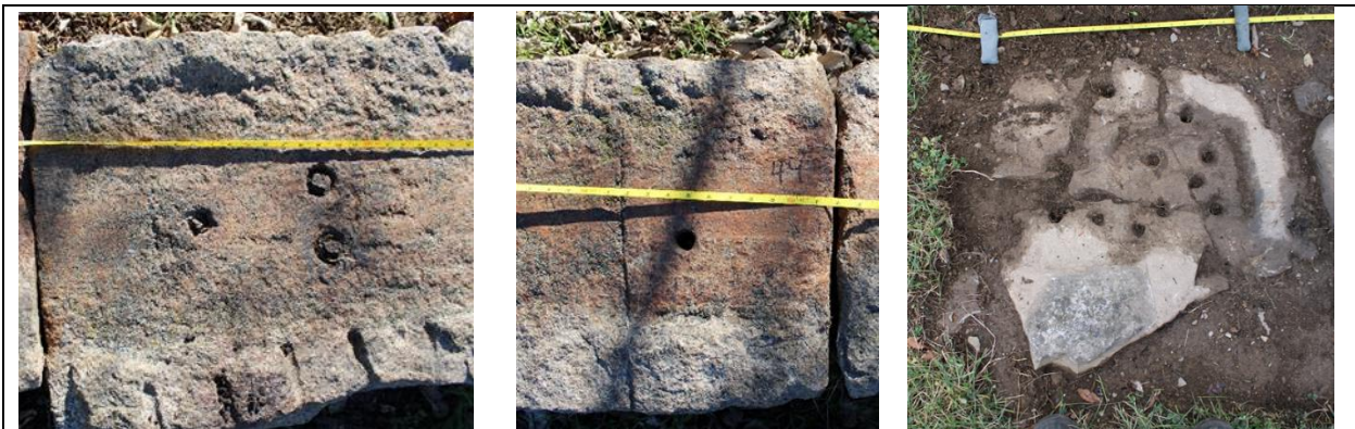
Figure 14. Spike holes for Rail Type 4: A) Two spike holes with square spikes on each side of a rail wear mark, B) Single spike hole on side of a rail wear mark; and C) multiple spike holes with no apparent pattern.
