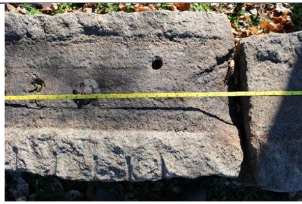
Figure 11. Narrow smoothed wear mark in chiseled groove that is created by abrasion of steel on stone.
