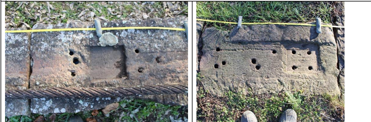
Figure 15. A) Two spike holes (for Rail Type 4) on each side of a rail wear mark adjacent to a chiseled box cut. A) Large diameter single spike hole for Rail Types 1, 2, and 5 between spike hole set. B) Two spike holes set within a chiseled box cut.
