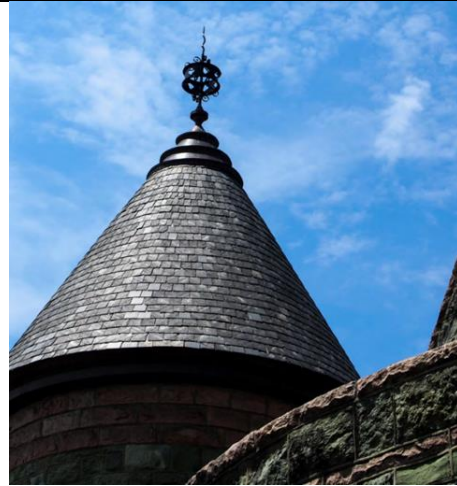
Figure 3. Roof of slate
