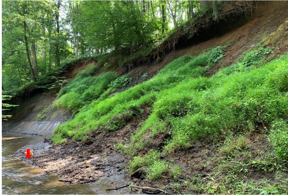
Figure 5. POI-2: Exposure just east of Boundary Road at Big Brook, Colts Neck, NJ. The red arrow points to a bucket that indicates the approximate location of this cliff in the 1970’s as remembered by J. Brown. It gives an idea of the degree of erosion and why study of Coastal Plain exposures are so challenging. The area above the arrow is highlighted in Figure 6. Photo facing southeast; by Justin Andell, RVCC.
