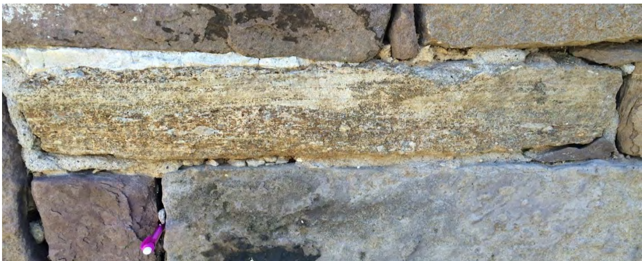
Figure 8: Brick at Prallsville Mills showing coarse pebbles down-cutting a sandy unit with pencil as scale (photo taken by
