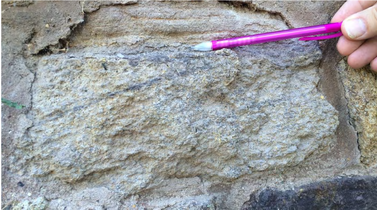
Figure 9: Brick at Prallsville Mills showing cross-bedding with pencil as scale (photo taken by F. Rea).
