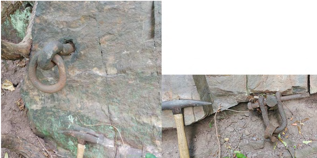
Figure 10: Weathered large metallic rings embedded in rock face that parallels the canal towpath.
