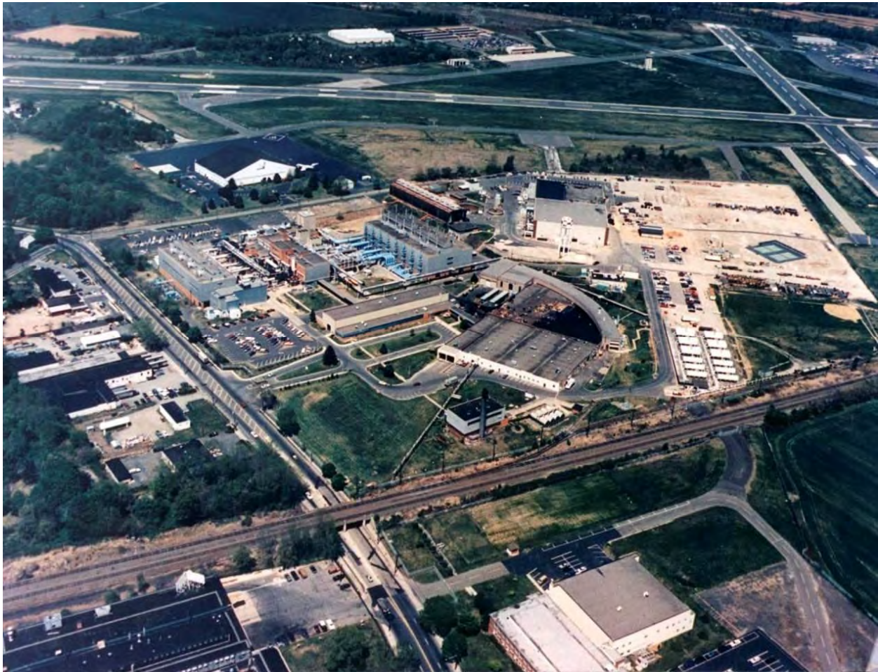
Figure 2: Air photograph of the former Naval Air Warfare Center.
