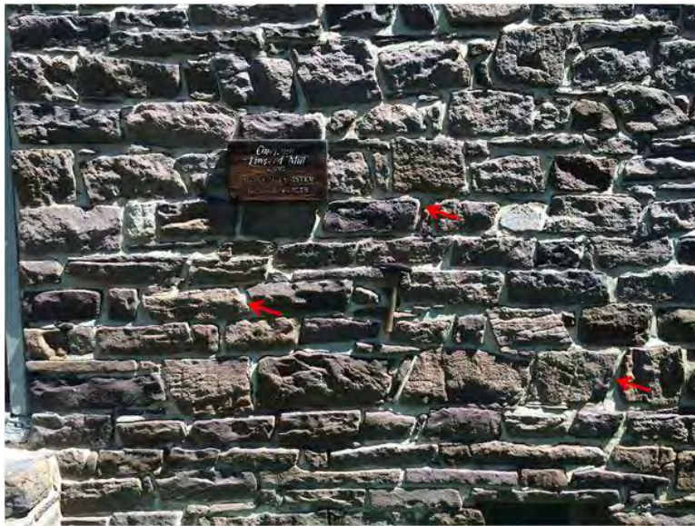
Figure 7: The original Linseed Mill building stone showing similar fracture patterns in the building stone with hammer for scale (Photo by F. Rea).
