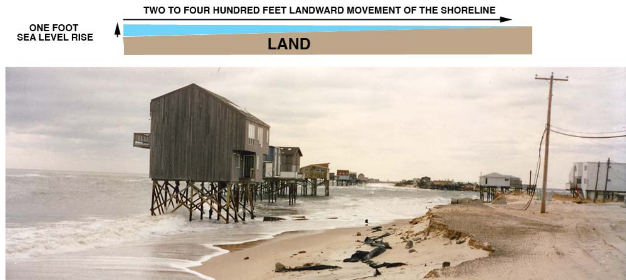
Figure 14. Effect of sea level rise on fixed structures. Top. On gently sloping sandy coasts a sea level rise of one foot can result in an inland translation of the shoreline of 200-400 feet. Bottom. The resulting erosion will eventually place elevated structures in the surf zone.
