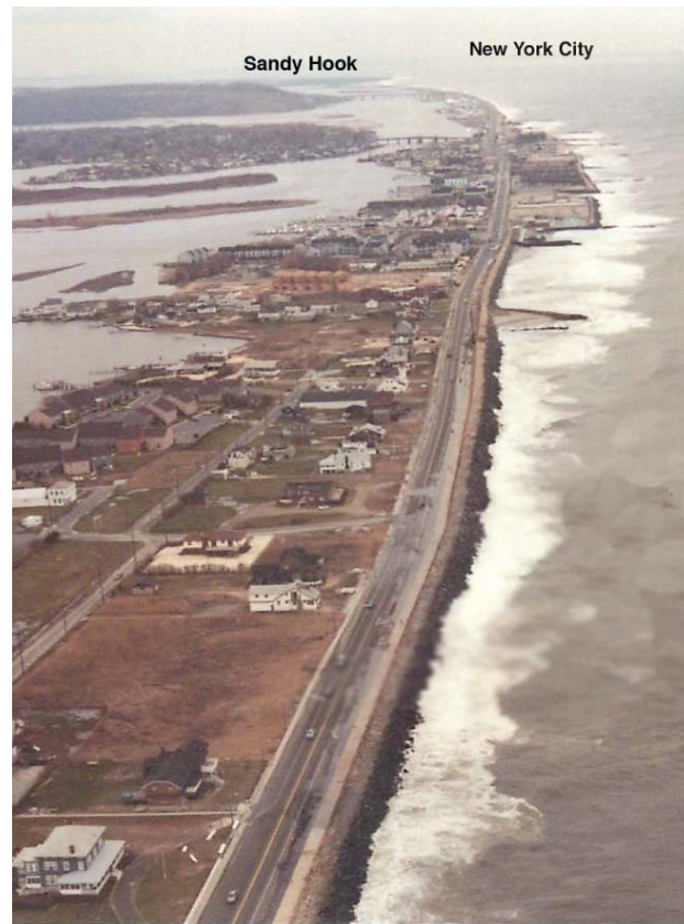
Figure 10. Seawalls and groins along the heavily engineered coast of northern New Jersey.
