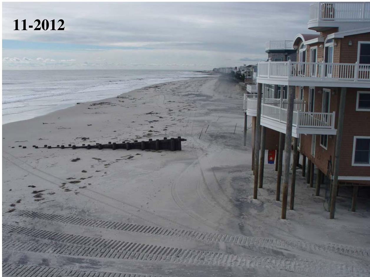
Figure 3C. Following Sandy (Nov 5 th ) the beach was flat and extended straight across the island to the bay. The vast majority of the dunes and everything placed under the buildings were removed and deposited landward. A CRC colleague's family home had debris (including a boat on its trailer) piled into the double garage to the floor joists and very little of it was theirs. Note the dune remnant in the distance that served a pair of homeowners extremely well because their landscaping was still intact. (photo-CRC, 2012)
