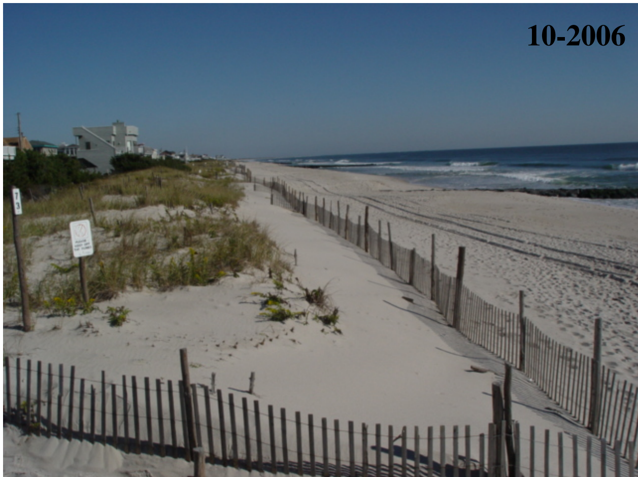
Figure 2A. In 2006, prior to the USACE project, the dunes were inconsistent in elevation and width. The low areas at pedestrian access paths were points where Hurricane Sandy's waves may have been able to penetrate and move sand and water landward. (photo-CRC, 2006)
