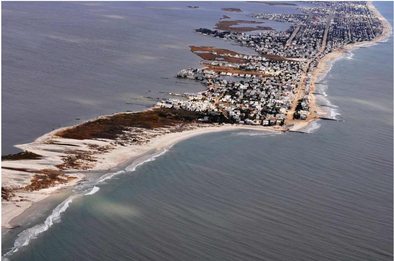
Figure 4A. Five days after Hurricane Sandy the CRC had the entire NJ coast flown yielding this photograph of the overwash and dune erosion in the Forsythe Wildlife Refuge plus the chaos that was existing on the Holgate section of Long Beach Township. In the upper middle right is a white patch of sand that represents one of the many overwash fans deposited on an undeveloped part of the island. The yellow sand is the fill material originally brought in to fill under the oceanfront homes and provide additional lot elevation. This was being moved back onto the beach. (photo-T. Kingston, 2012)
