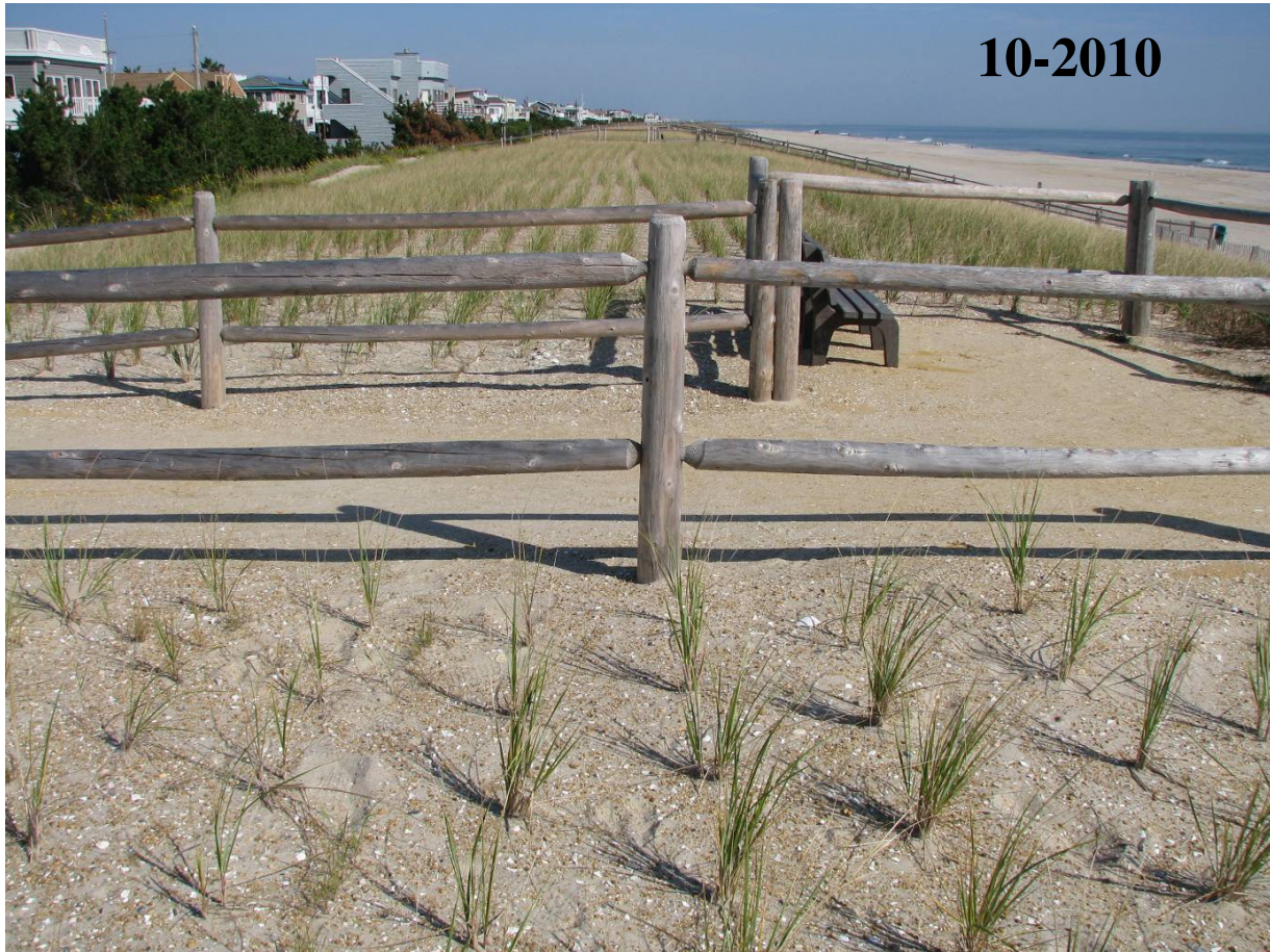
Figure 2B. In 2010, prior to Hurricane Sandy this view to the north shows the new, consistent elevation dune with its plants in place. The 22-foot crest elevation was not so great as to block water views as owners initially feared. This was because many dune crests approached 20 feet in elevation if only in spots. Note the vastly greater dune width after the project. (photo-CRC, 2010)
