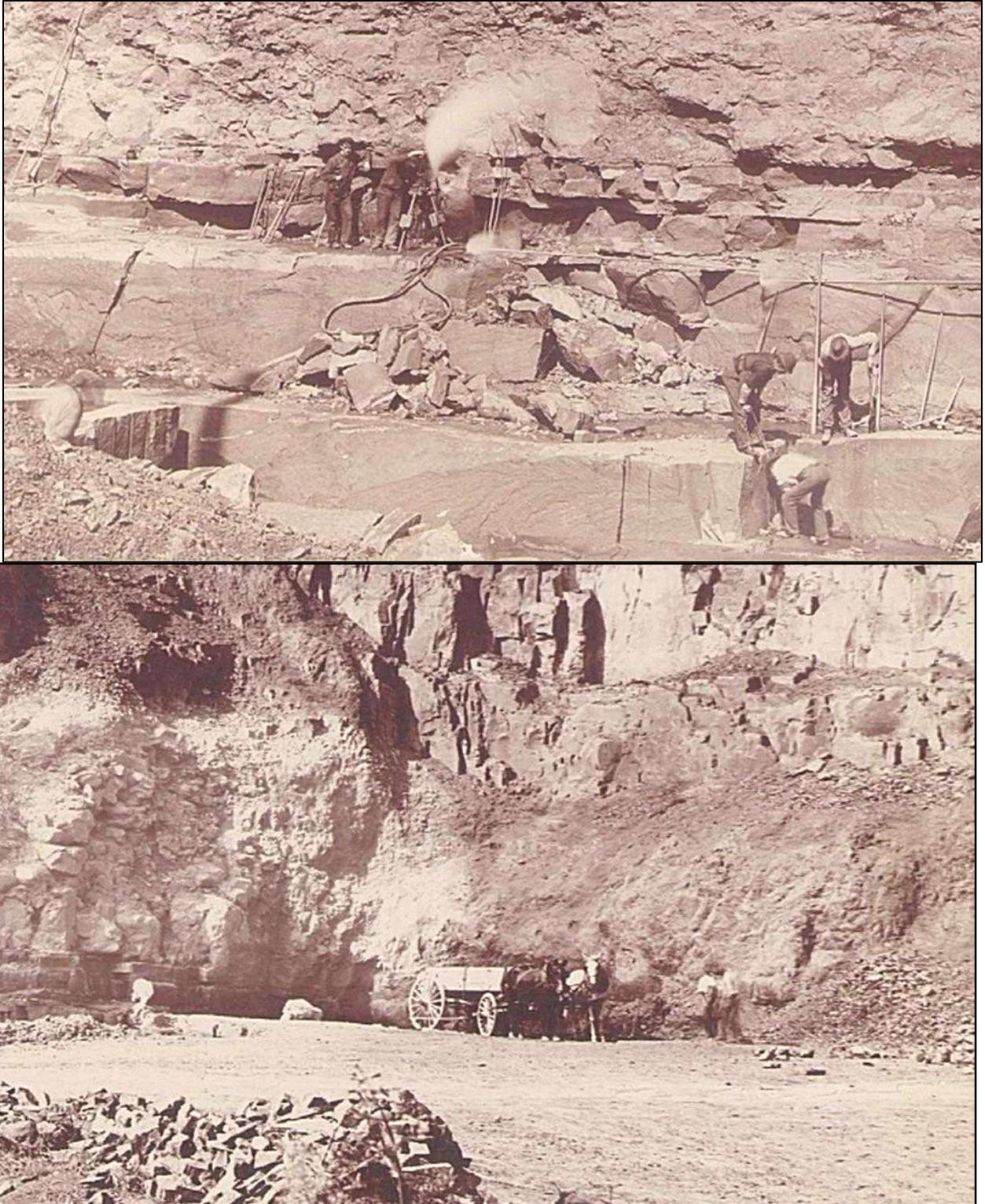
**Figure 6.** Montclair brownstone quarry operations circa 1905. A. Wedge and feather quarrying of blocks with a steam drill on one bench drilling vertical holes and a crew on another bench working on horizontal holes. B. Wagon team in the Montclair brownstone quarry.
