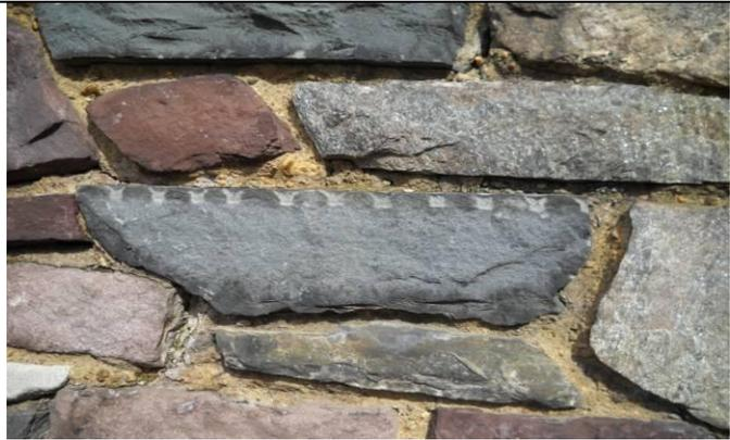
Figure ft-4a Mining features, Pin and feather rock breaking technique in dark sandstone.
