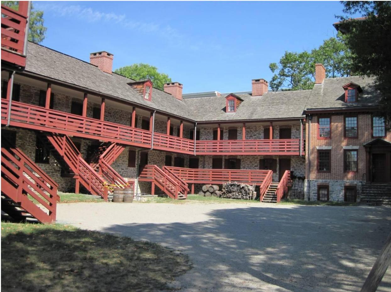
Figure ft-5. Old Trenton Barracks. Most stone work is original. Section between two wood barrels and five wood barrels are not original. Brick façade is not original.
