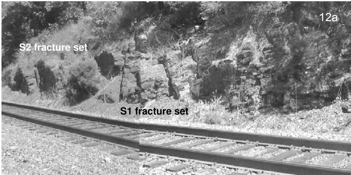
Figure 12a. S2 fracture set terminating against S1 fractures in red mudstone cropping out along a railroad cut in Hopewell Township, Mercer County.
